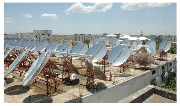
Figure 16: Roof Top Installation of Solar Concentrator Dishes at an Educational Institute
